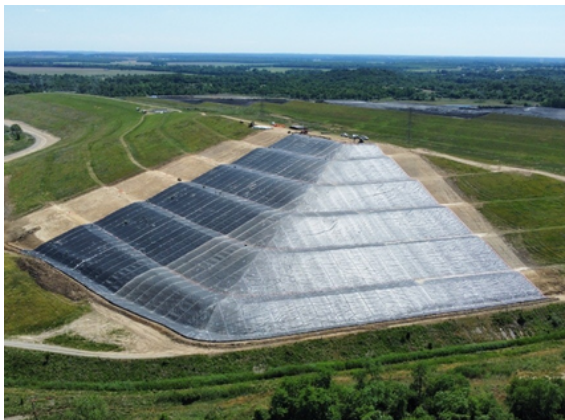
WILSON STATION LANDFILL WITH GEO-SYNTHETIC MEMBRANE COVERED WITH TURF
